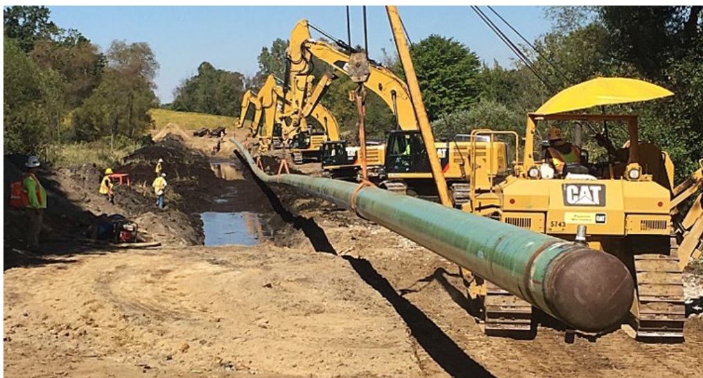
Figure 17: Illustrative pipeline installation 41
